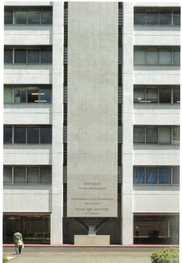
Left: Research Office Twin Towers, Tokyo (2002). Utilizes a seismic isolation system
